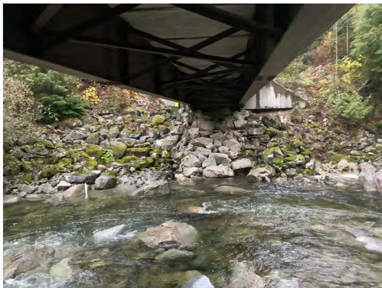
Left Bank Abutment when facing downstream
