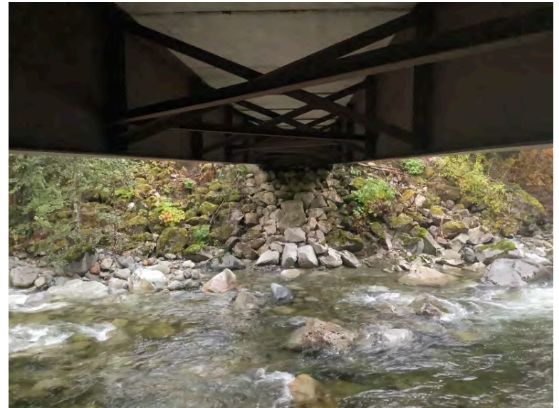
Right Bank Abutment when facing downstream
